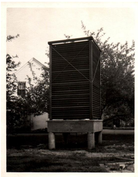
May 7, 1939 building site for 17 Orchard Lane
